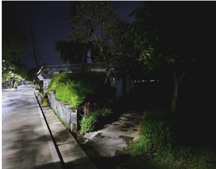
Figure 6. Non-functioning Lighting in the Toilet Area at Lapangan Renon (Night Condition) Source: Lesmana (2026)
